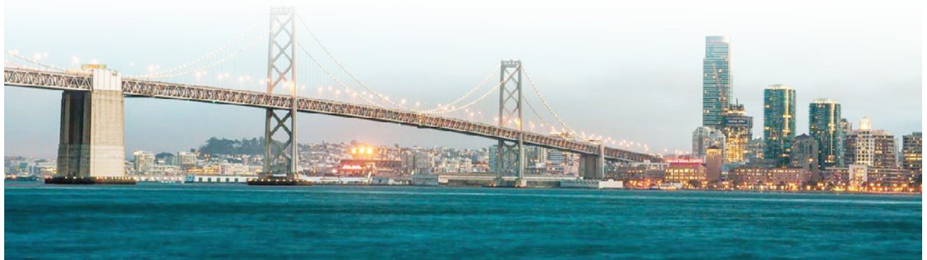
Figure 2.1. The concrete pylons of the San Francisco Bay Bridge counter the weight of the suspension bridge and vehicles by simply being heavier. https://www.pexels.com .
