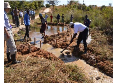
Construction of small-scale irrigation facilities by farmers
