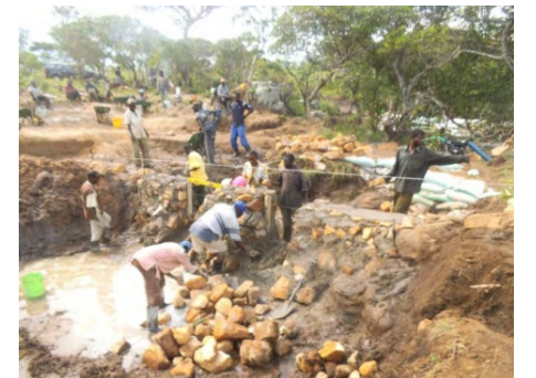
Construction of permanent weirs by farmers, by stonework
