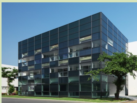
Fig. T1-1 Building facade
