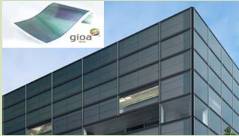
Fig. T1-4 BIPV by the organic thin film
