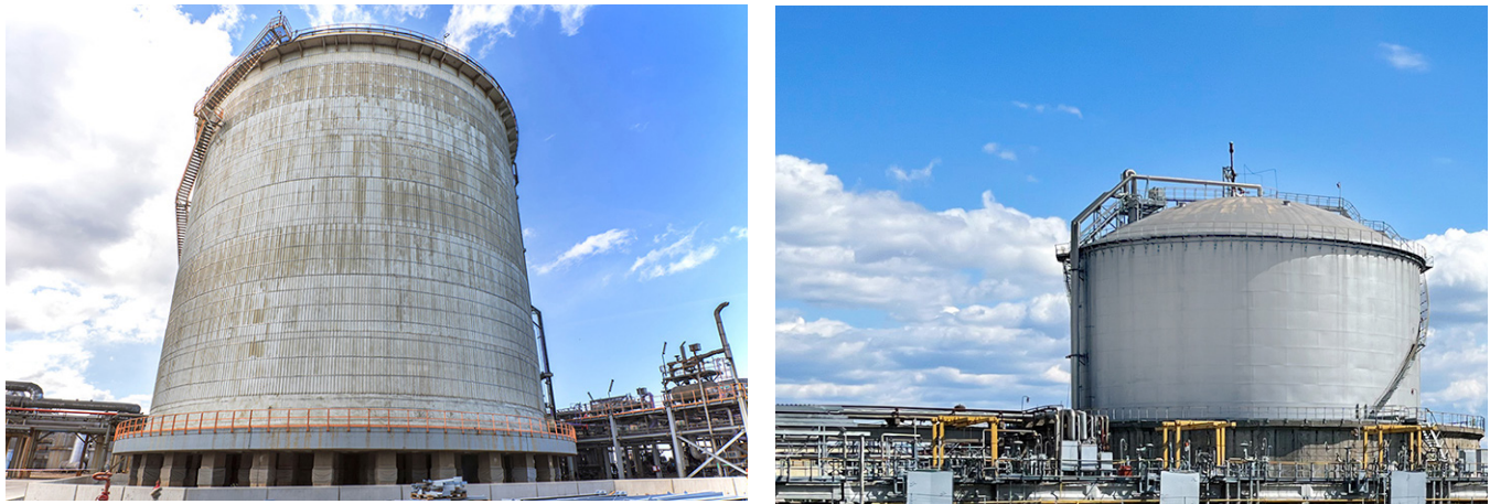
Figure 4-5. Refrigerated ammonia storage tanks.
