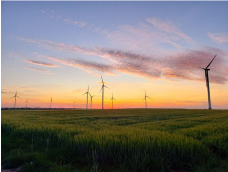
Figure 3-5. Green Ammonia production depends upon the continued build-out of renewable energy production capacity. (credit: Ann-Kathrin Merz)
