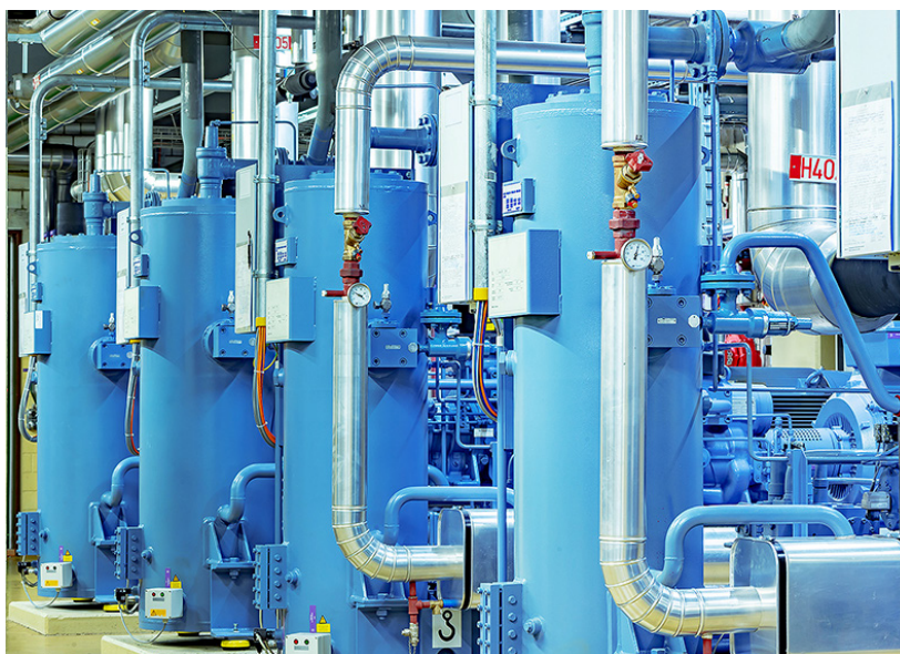
Figure 5-5. Industrial ammonia refrigeration system 65
