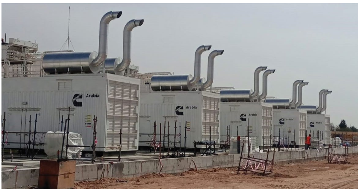
Fig. 3.1-2. Multiple diesel generator sets, of the kind used to provide reliable backup power at data centers.
