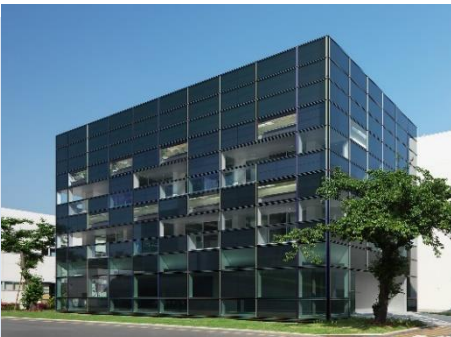
<Side wall> reference: https://www.taisei.co.jp/about_us/wn/2014/140616_3948.html (大成建設HP)
