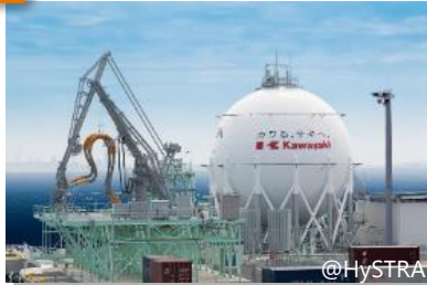
Storage Tank at Hy touch Kobe: 2,500m 3
