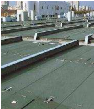
Lid of Sewerage Bureau (tie-up with Tokyo metropolitan government)
