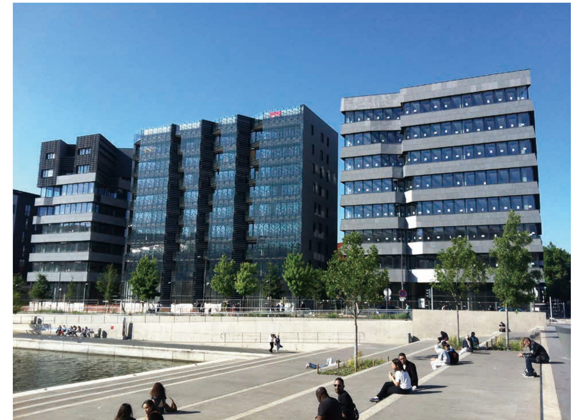
Positive energy building “HIKARI”
